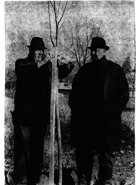
TYING LOOSE ENDS — With completion of its 36-inch pipeline across Oakland Township, Michigan Consolidated Gas Co. is fulfilling its agreement with the township to replace 80 trees removed during construction on Inwood, Hadden and Gunn roads. Norbert M. Karmann (left), forestry expert with the utility, ties one of the newly-planted maple trees to a stake as Raymond Alt, Oakland Township highway commissioner, gives his approval.
