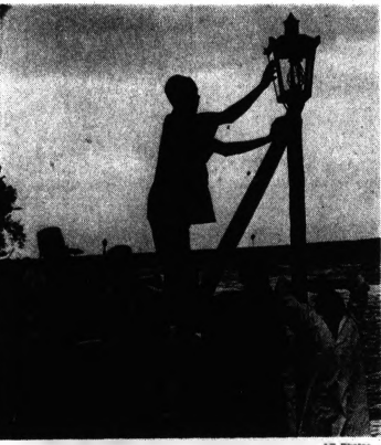
JOB IN JEOPARDY — A lamplighter places a kerosene lamp in position at the quayside at Lamu, Kenya. His job soon will be discontinued with the advent of electricity.
