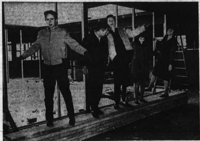
NEW CONSTRUCTION—Balancing on materials at the construction site at Pontiac Northern High School are (from left) students Rick MacAuley of 3374 Simmons Road, Alex
