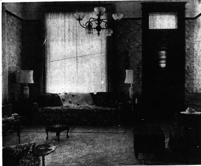
Frosted Globes Found On Original Gas Chandelier Now Electrified
