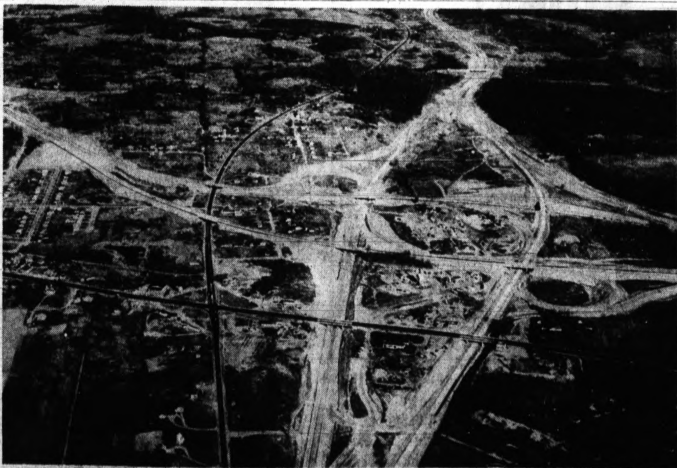
INTERCHANGE EAST OF BRIGHTON — This aerial photo, looking north, shows the interchange of I-96 and U.S. 23 freeways east of Brighton. The huge traffic complex, spread over 175 acres of land, is one of the largest interchanges in the world. It will be completed next year when U.S. 23 (north-south) freeway is opened to traffic. The $5.8-million project will eliminate part of a major traffic bottleneck at the intersection of U.S. 16 and U.S. 23—the back-log roads which cross the lower part of the photo. It also will remove a major detour for through traffic on I-96.
