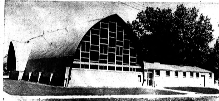
SANCTUARY COMPLETED —The new addition to St. James Missionary Baptist Church, 345 Bagley will be dedicated at 3 p.m. tomorrow. Rev. T. H. Holt, pastor of greater Mt. Calvary Baptist Church, will conduct the service.
