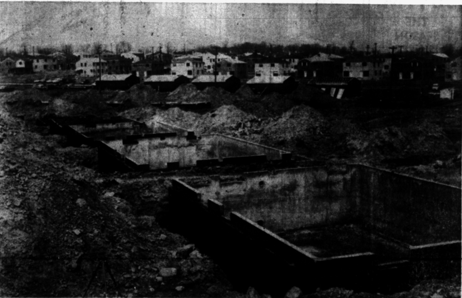
STAGES OF BUILDING — An over-all picture showing the development of the new housing on the south side of East Boulevard reveals the different stages of building in process. At the base of the hill, several houses are nearing completion. Also visible are
