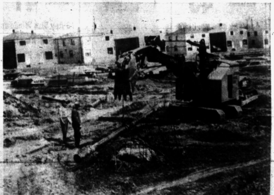
CRANES SWING INTO ACTION — Part of the earth-preparing scene going on today out at the new East Boulevard development include large cranes at work placing sewer lines and basement forms.
