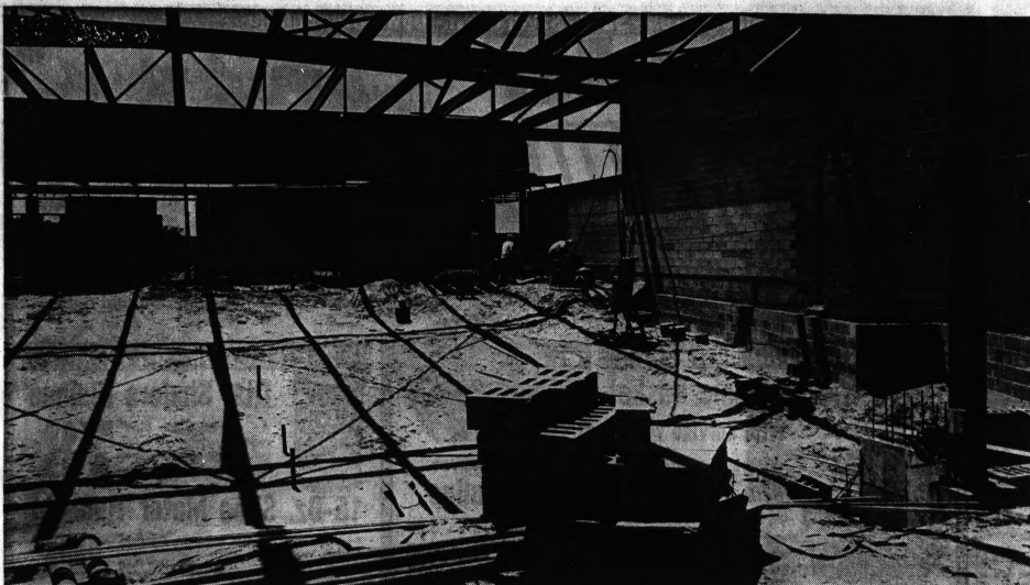
NEW AUDITORIUM — School officials are hopeful that construction work on the new auditorium for Rochester High School will be completed in time for the opening of the second semester of the coming school year. The auditorium is part of a
