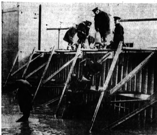
FIGHTING THE OHIO —Fireman reinforce a flood wall in downtown Louisville, Ky., in hopes of stopping the mighty Ohio River. The river stood at 18 feet above flood stage
