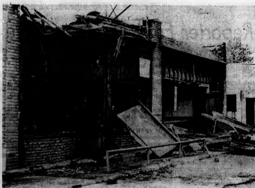
RESTAURANT DESTROYED — Only a few charred timbers and cement block walls were left of Vincent's Dining Room, a Keego Harbor establishment operating at 3049 Orchard Lake for nearly 30 years, after a
