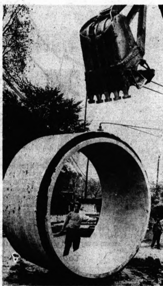
GIANT'S RING — Better watch out, Mister, a slip of that cable and it could mean pancake feet. A single section of drain pipe such as this weighs 15 tons. Here it is being lifted into the waiting ditch where Otis Avenue in Hazel Park used to be.
