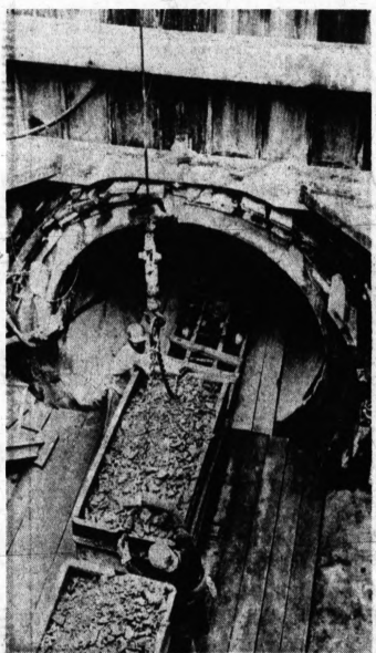
"HOOK 'ER UP" — Hooks are attached to the clay-filled bin so that a huge crane overhead can lift it onto dump trucks waiting at street level above. The clay is then hauled off to be used as fill somewhere else on the mammoth project worming its way through 12 communities.
