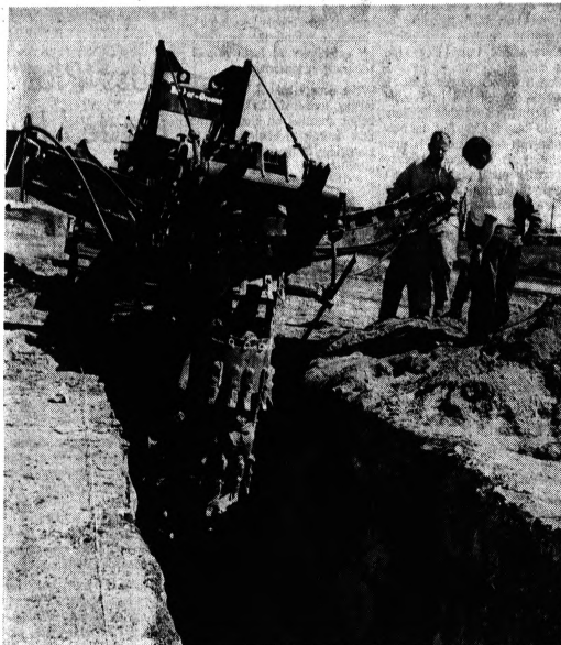
READY FOR MAINS — Trenching machines set to burrow into the ground an even seven feet are being utilized by crews laying water mains in Waterford Township. The task of laying 135 miles of water main began last week. Mains range in size from 6 to 36 inches
