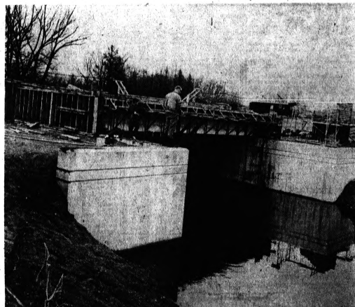
NEW BRIDGE — The five-lane bridge under construction over the Clinton River west of Crescent Lake Road is scheduled for completion by June 15. A major phase of the M59 road widening project, the new bridge replaces the former two-lane bridge which was
