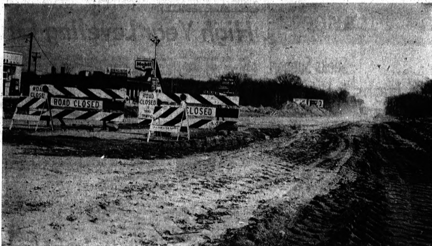
M59 CONSTRUCTION — This photo taken at M59 and Pontiac Lake Road looking southeast shows a portion of the 3.4-mile M59 construction zone between Elizabeth Lake and Airport roads. The $1.3-million State Highway Department project will widen the existing two-lane road to five lanes. Work started in January and the road is scheduled to be open to through traffic by Labor Day. Local traffic only is permitted now. Paving is slated to begin
