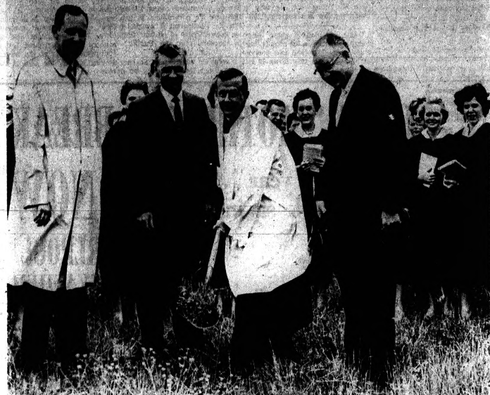
BREAK GROUND FOR CHURCH — In festivities following yesterday's morning worship service ground was broken for the new Calvary Lutheran Church on a site just north of the Clarkson village limits, west of M15. Taking part in the ceremonies were, from left, E. W. O'Brien, of the Waterford Construction Co., general contractor; Martin Gustafson, chairman of the building committee; Paul A. Johns, pastor, and T. Neel Eubank of Flint, architect. The congregation, organized Jan. 2, 1961, now numbers 108 adult members and 117 children.
