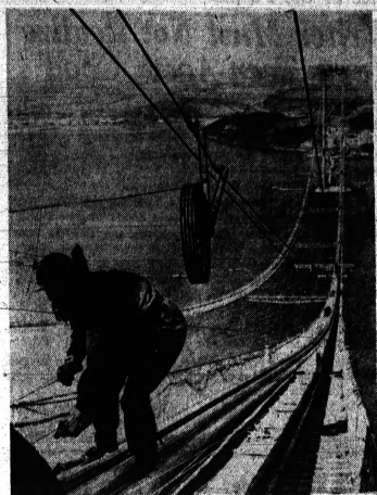
HIGH WIRE ACT — Workman Richard Stewart inches up a catwalk alongside the main cable of Scotland's new Forth Road Bridge which spans the Firth of Forth between North and South Queensferry in West Lothian. The spinning wheel in the background stretches cables between supports. This will be the largest suspension bridge in Europe and is expected to open traffic in mid-1963.
