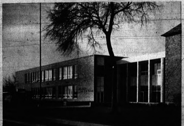
Jefferson Junior High - refurbished inside and out.
