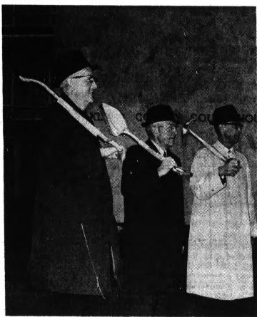
COUNTY GROUND-BREAKERS—Heading in to the shelter of the Oakland County Courthouse after breaking ground yesterday in a driving rain for the $3-million John A. MacDonald East Wing of the courthouse are the three members of the County Building Authority. From left are Harry L. Lapham, assistant vice president of the National Bank of Detroit; Robert M. Critchfield, retired GM vice president; and Milo J. Cross, president of Pontiac State Bank. Some 75 governmental officials and civic leaders turned out for the ceremony.
