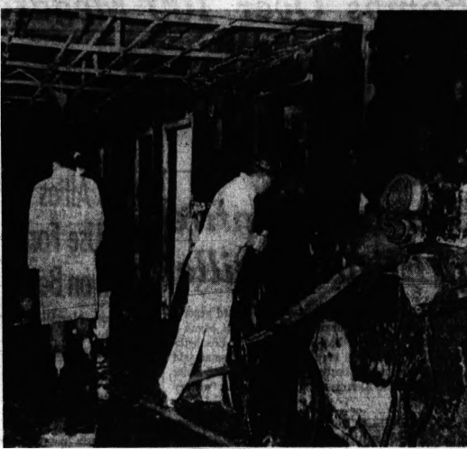
INSPECT FIRE RUINS — Firemen and officials inspect a burned hallway on the ninth floor of Hartford Hospital after fire killed 15 persons Friday. More than 100 were trapped in hospital.
