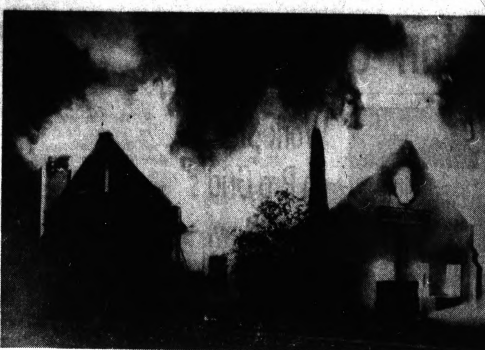
CHURCH DESTROYED—The First Baptist Church of Johnson City, Tex., was destroyed last night by a fire of undetermined origin.
