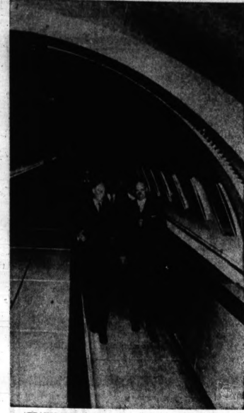
"TRAVOLATOR." BRITAIN'S MOVING SIDEWALK — Sir Edmund Stockdale, right, Lord Mayor of London, joins officials for a ride on the "Travolator," Europe's first moving pavement. It runs 104 yards between two subway stations. Belt tracks move on 3,904 wheels up to 180 feet a minute.
