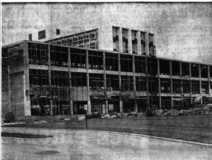
EAST WING —After being delayed some 30 days by severe winter weather, construction on the $3.1-million east wing of the Oakland County Courthouse now is progressing, with completion scheduled for April 8, 1968. General contractor for the 85,000-square-foot wing is Barton-Malow Co. of Oak Park, and the architects are Odell, Hewlett and Luckenbach of Birmingham.
