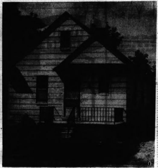
AFTER REMODELING —Now the little house at 28 West End has a bright new exterior, new storms and screens all around and an additional room on the back (which you can't see.) The little cement porch gives the front of the house a more graceful look. Federal Modernization did the work.
