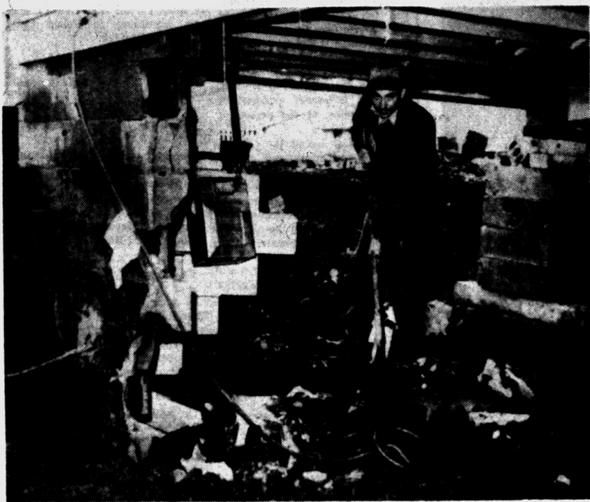
MISSING: ONE FOUNDATION — Harold Thacker of Chillicothe, Ohio pokes around gingerly trying to locate the basement floor in his new house. A flood swept away most of his basement walls. Approximately the same thing happened to 50 of 55 houses in the same subdivision. The column of blocks at right is emergency shoring to keep the house from collapsing.
