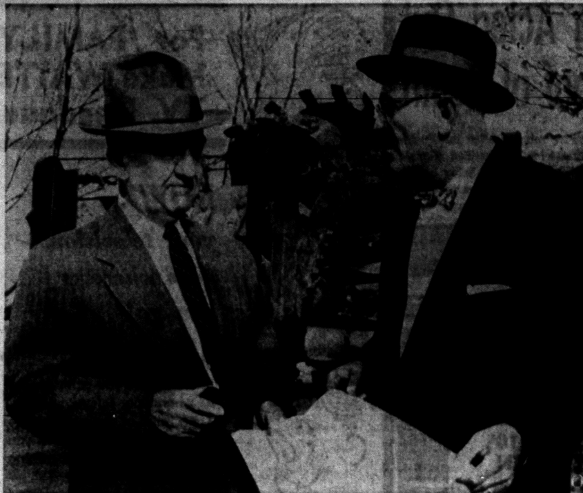
START MILFORD'S MAINS — Peter Ramsey, boss of construction of the $300,000 project to give Milford gas service, at right, and Charles R. Henderson, district manager out of Ann Arbor stand by the big "digger" that broke ground Monday. They are looking over master blueprint of mains' routings.
