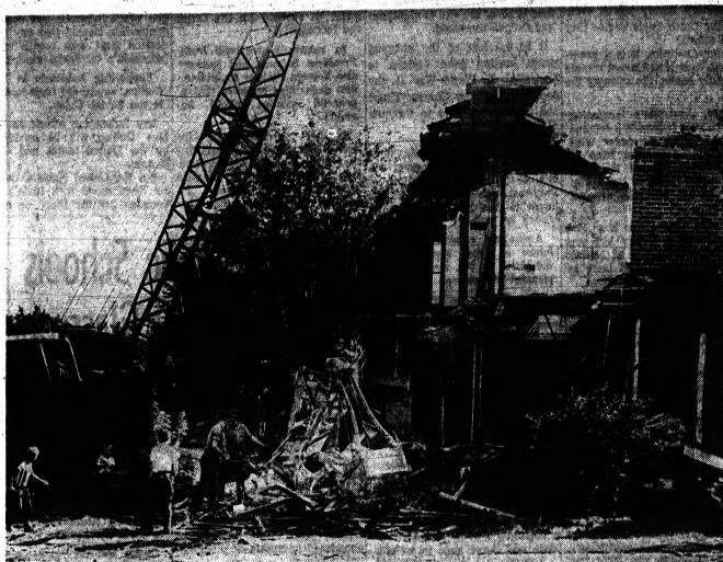
URBAN CLEARANCE UNDER WAY —With final approval of Pontiac's first major urban renewal clearance contract at a Sept. 5, 1961 City Commission meeting, demolition work began in a renewal area. Pictured are crew members of Dore Wrecking Co.
