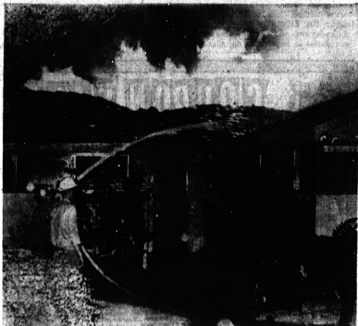
FUTILE BATTLE —Firemen spray water on roof of a home in Montecito, Calif., a Santa Barbara suburb, in a vain effort to save the expensive structure from flames. A raging brush fire swept through the area during the night.
