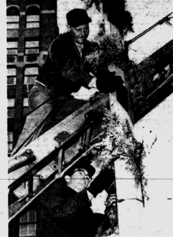
DECORATING STREETS — Two city workers wrap around a Huron street light pole one of the Downtown Merchant Assn's ever-green festoons. Helping get downtown set for Christmas are electrical employees Norman McCormick (top) and Richard Sullivan. The association's giant Christmas tree will go up Nov. 30 at the corner of Saginaw street and Oakland avenue.
