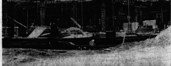
HUDSON EXPANSION — Construction workers go about their chores in erecting a new $2.4-million addition to the J. L. Hudson Co. store at the Pontiac Mall. About 200,000 square feet of floor space will be added to the present facility, making it a full-line department store. Completion of the expansion is earmarked for 1967.
