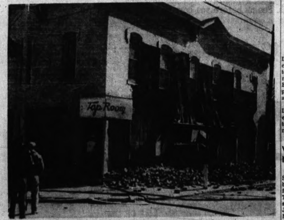
BLAST SCENE — An explosion shook the 100-year-old Millington Hotel yesterday but none of the 36 occupants were seriously injured. The exterior of the building is shown here with one wall crumbled. Leaking gasoline is believed to have been the cause. Millington is on M15, seven miles south of Vassar.
