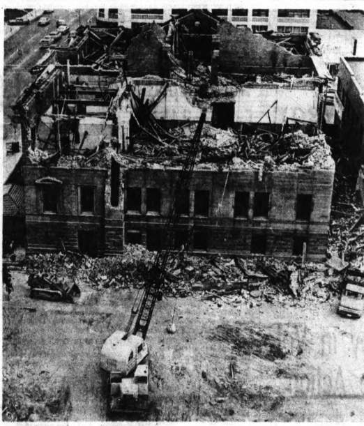
CRUMBLING COURTHOUSE — From top of the Riker Building, corner Wayne and Huron streets, the camera looks into the vanishing Old Courthouse. The large room laid open in front was a courtroom, with a judge's chambers at left. Chambers and court are separated by a wall and white-columned portico still standing where once the judge's bench was.
