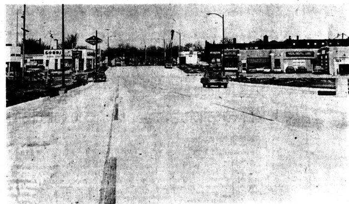
WIDE, WIDE TRACK — The final stretch of Pontiac's multi-lane loop road, offering five lanes that encompass the downtown area, opened to traffic yesterday. The final stretch runs from West Huron to South Saginaw. These first cars head south from West Lawrence on the final leg.
