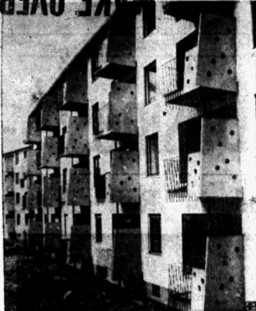
SWISS CHEESE BLINDS - Perforated sunshades are conspicuous on balconies of new apartment houses in the U. S. sector of West Berlin. Holes permit limited vision.
