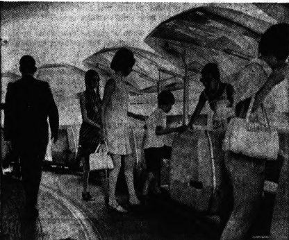
Passengers for "PeopleMover" cars, right, step from a moving, 90-foot-diameter ring on which they're standing, into the cars. Ring moves at a steady, synchronized-with-the-cars 1 1/2 m.p.h.
