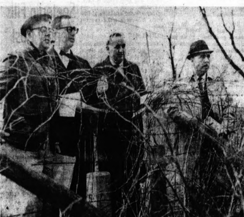
INSPECT SITE — Looking across part of 3,800 acres of Northfield Township land proposed as the site for the $45 million National Accelerator Laboratory is Atomic Energy Commission site selection team members (from left) Enzo DeRenzi,
