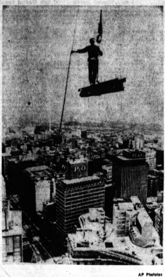
ON THE BEAM — Steel Shelton dangles in space on a load of steel girders, 500 feet above a street in Sydney, Australia. He directed crane operations during completion of a building that will tower 440 feet above the main thoroughfare.
