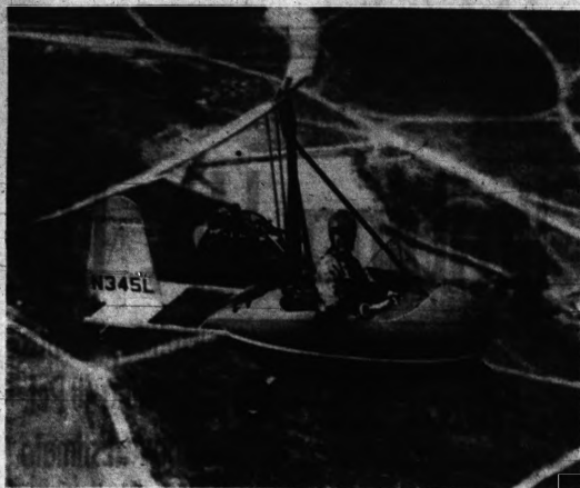
'NO TRAFFIC UP HERE' — Herman Saeftel, 31, flies over rural area near San Diego, Calif., in his Skycopter, which has pusher engine and nonpowered rotor. He said he has quit his draftsman's job to turn out the craft in home-assembly kits. A shooter like this certainly avoids Fourth of July traffic ground problems.
