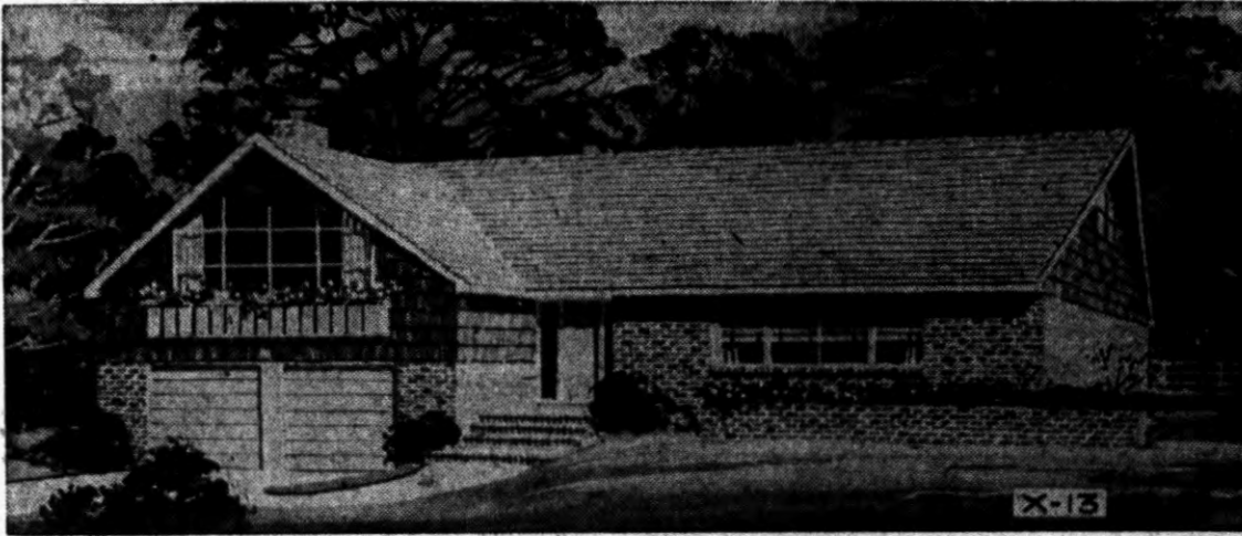
NEW DESIGN IDEA — Brick veneer and wood shingles are used as exterior materials for this house which combines the structural technique of split level planning with ranch design. The studio is over the garage.
