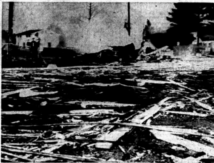
TWO BUILDINGS RAZED — Two fireworks storage buildings occupied the space shown above, covered with smoking debris, in Portland, Ore. The buildings blew up at 1:45 a.m. today, for reasons not immediately determined. Houses and stores in the area suffered heavy damage from the blast.
