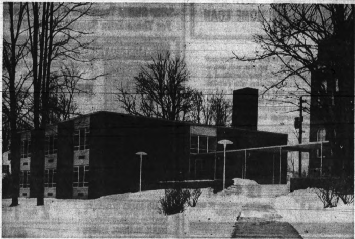
OPENS MONDAY — Work should be completed this week on the new two-story addition to Romeo Junior High School. Contained in the brick building are four classrooms and laboratories on the ground level and two science laboratories and two classrooms on the floor above. The structure also houses a
