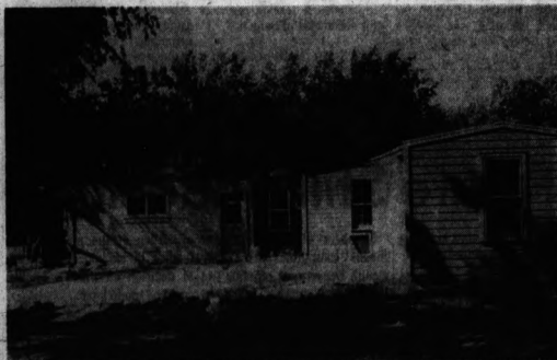
MEANWHILE QUARTERS—Construction crew shacks serve as quarters for St. Augustine's House while the new house is being built. Donated recently by Darin and Armstrong, a Detroit construction firm, the shacks
