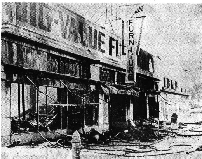
GUTTED — The fire and smoke-blackened store front of Big Value Furniture Discounters, 47-55 S. Saginaw, shows the intensity of the blaze that swept through the building last night. A fire wall kept the blaze from spreading to the adjacent supermarket.
