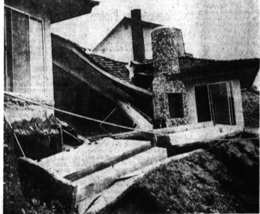
GOING, GOING, ALMOST GONE — This hillside home in Encino, Calif., is only one of a number that are slowly collapsing as the result of landslides in southern California from the heavy rains. The state had more rain today and a new 6-inch snowfall blanketed the Midwest.
