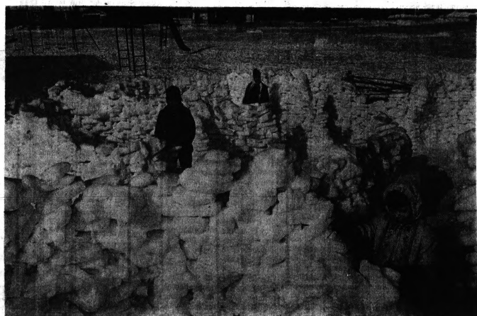
"THOSE WALLS SHOULD HOLD!"—Lambert school students Jeff Aiken, Laurin Graves (middle) and Sandra Eggert check the house they and other junior home builders constructed on the playground next to their Waterford Township school. With slabs of crusted snow several inches thick, they created the structure which will have running water at the first thaw.
