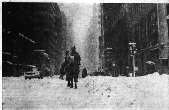
POOR ADVERTISEMENT —The heart of New York City's advertising district, Madison Avenue, was a poor advertisement for the city this morning as pedestrians took to the middle of the street to plow their way through the heavy snow. There was little to fear from automobiles, which were, in large part, snowed in at home. It was the third knockout blow by the city's worst winter in 80 years.
