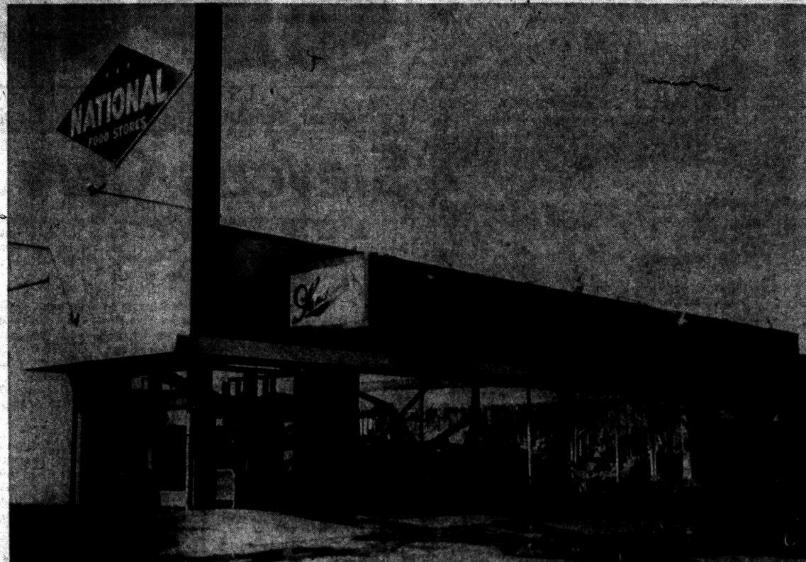
GUTTED BY BLAZE — A loss of $200,000 is estimated by Farmington Fire Chief Joseph DeVriendt as the result of a flash fire which swept through the National supermarket at 10-Mile and Orchard Lake roads Saturday evening. The store manager was injured when he tried to extinguish the flames before arrival of five area fire departments. It took them better than an hour to arrest the blaze which was still smoldering late Sunday.
