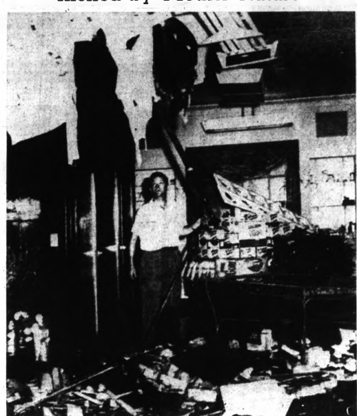
NOT SO FLOWERY — Jacob Hoogendorn surveys damage to his flower shop in Kalamazoo following Wednesday's violent storm. A funnel toppled the chimney onto the roof and the bricks crashed through to the ground floor. A Kalamazoo theater also was damaged and telephones were put out of service.
