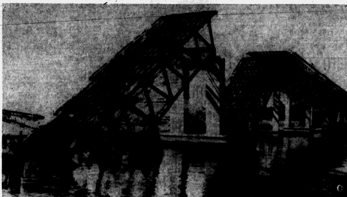
TWO SECTIONS FALL — Twisted steel of two sections of the nearly completed new Second Narrows Bridge near Vancouver, B. C., lies in Burrard Inlet after collapsing with a thunderous roar Tuesday and killing at least 16 workmen. Two men are missing and 22 were injured. The $16,000,000 span, replacing the old Second Narrows Bridge, was to have been completed this year.
