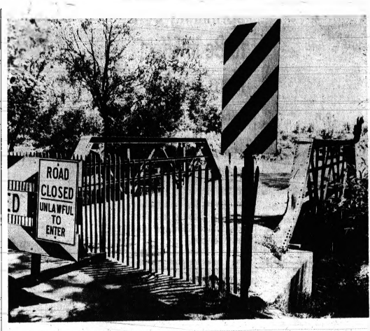
TO BE REPLACED — Bids will be taken July 11 by the Oakland County Road Commission for construction of a new bridge to replace this "one-way" span currently out of use on Pontiac Lake Road west of Highland Road. Work on this and two similar bridges on Dutton and Avon roads in Avon Township is expected to begin Aug. 1. Ten such bridges too narrow for more than one car are to be replaced this year with the help of $212,000 in federal matching funds.
