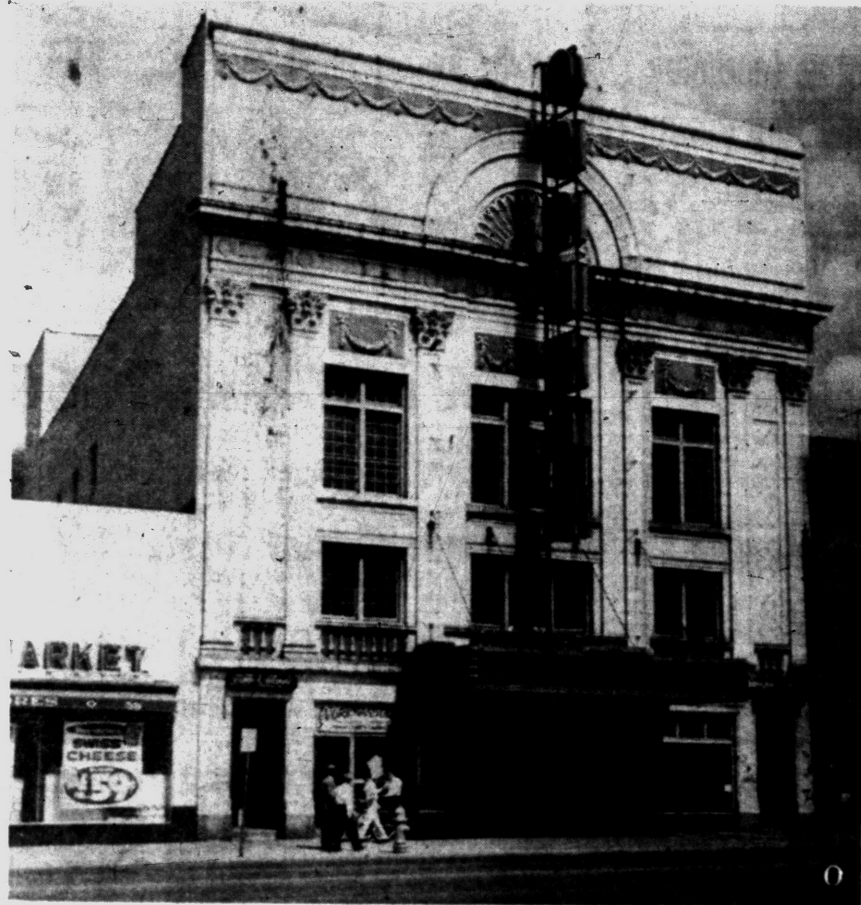
COMING DOWN — Take a last look at the Orpheum Theater on S. Saginaw street, north of Auburn avenue. After several years of idleness, the 34-year-old movie palace is being torn down to make room for a parking lot, the owner says.
