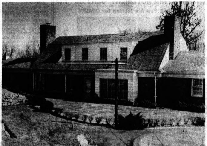
THE MARTIN HOUSE —It seems to snuggle down into the hill here, but appears to be perched high on a hill on the road side. The old-time brick is accented by gleaming white
