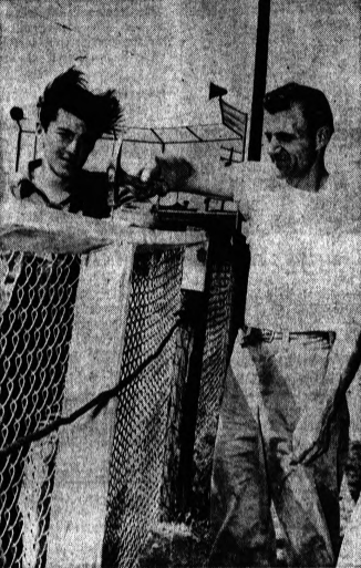
READYING BALL PARK —Waterford Township Cemetery and Parks Department crew members Dave Golt (left) and Alvin West are putting in a new section of fence all the Drayton ball park. This and several other fix-up projects were to be completed today. The recreation department will put the field in playing shape early next week.
