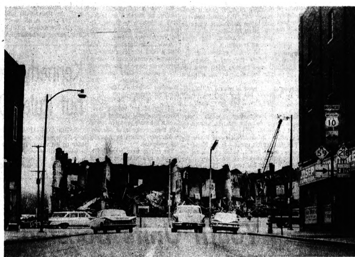
CLEARING WAY — The scene is changing at the east end of Orchard Lake Avenue. The buildings on the east side of Saginaw Street, just north of Auburn Avenue are being wrecked
