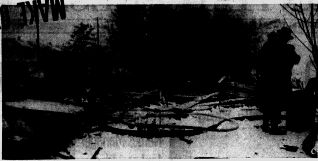
IT ONCE WAS A HOME — Police and fire officials above clamber through rubble left after an explosion leveled a four-room bungalow at 169 W. Columbia Ave. about 11:15 yesterday. No one was in the house, they said, after a search which indicated escaping gas may have caused the blast. Owners Leonard and Beatrice Gravitt, a retired couple, were informed of the loss in Florida, where they were vacationing.
