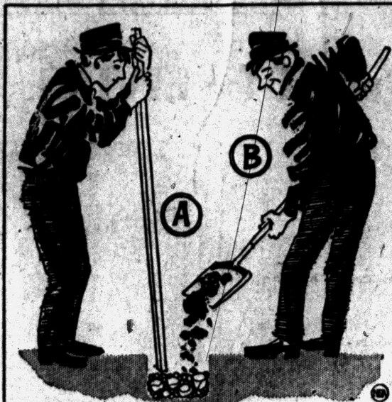
BLACK TOP REPAIRS —Large stones and gravel, well packed (A), make a good base for black top repairs with a commercial patching mix (B).
