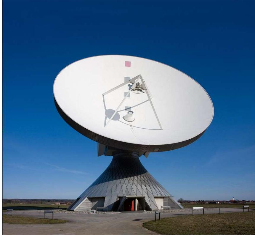
Figure 1.18: Parabolic dish reflector antenna [60]
