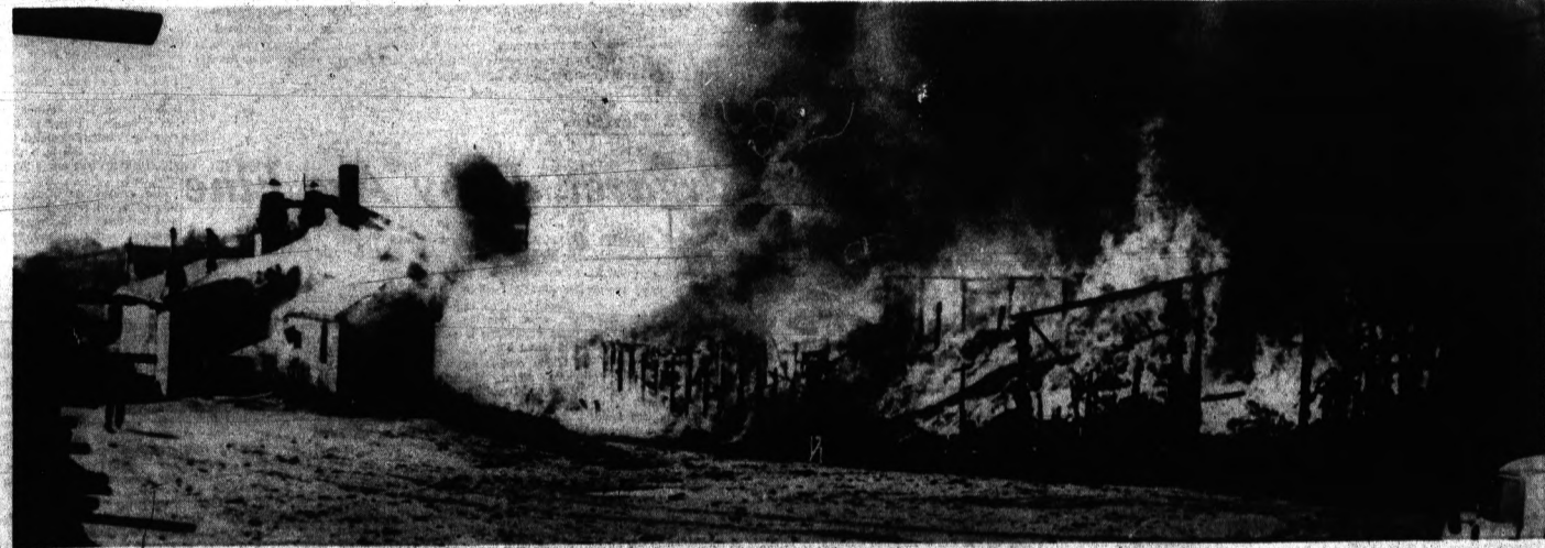
Roaring Out of Control, Flames Devour the Pontiac Millwork Co. and Spread to Adjoining Structures
