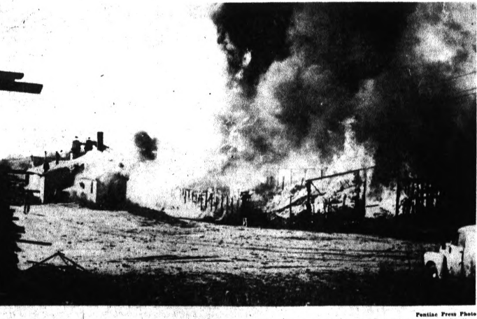
TOTALLY DESTROYED — Roaring out of control, flames enveloped the Pontiac Millwork Co. buildings at 2005 Pontiac Road in Pontiac Township. Firemen from six departments struggled to keep the fire from spreading to surrounding buildings, including a motel. The blaze started at 9:15 a.m. Shown here is the rear of the firm's buildings in the general area where the fire started.
